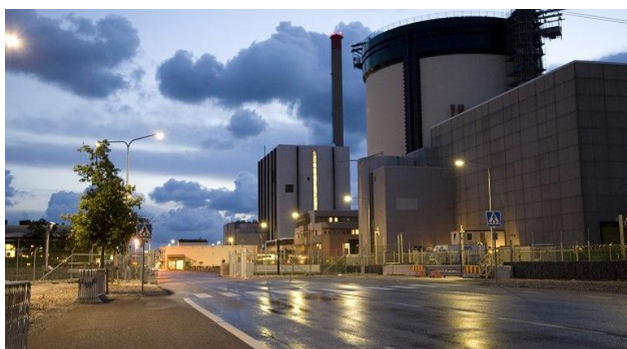
Figure 8. Ringhals nuclear reactor in Sweden, operated by Vattenfall [Courtesy of Vattenfall]
